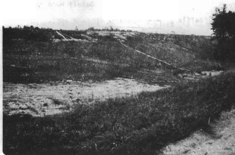
Flexible down drain - installed
